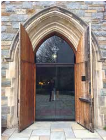
Western Avenue Glass Entry Doors
