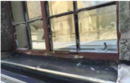
Glazing, Painting and Cleaning of Parish House Windows
