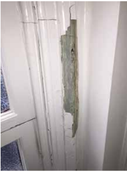
Interior "Old" Men's Bathroom
