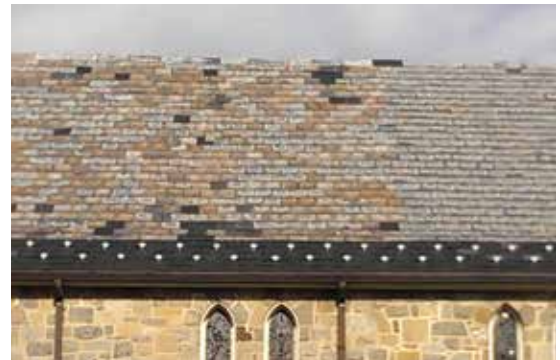
Nave Slate Roof
